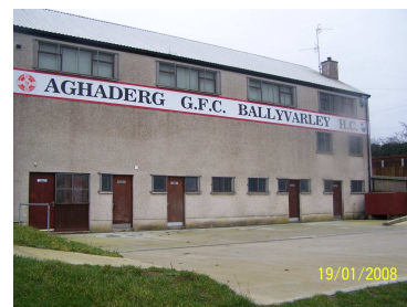
New Concrete To Front Of Dressing Rooms
